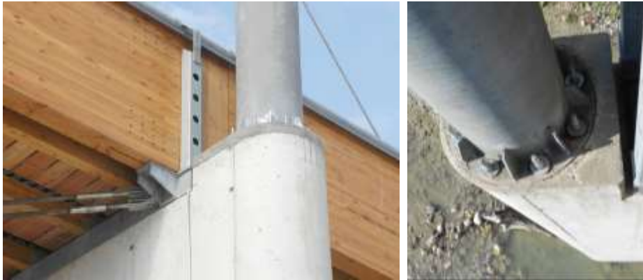
Figure A.2.15. Detail of the internal support made by reinforced concrete.
