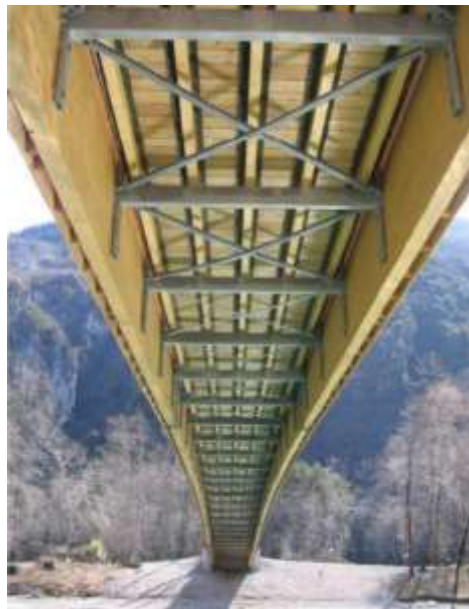
Figure A.1.6. View from above of the structural scheme of the deck.
