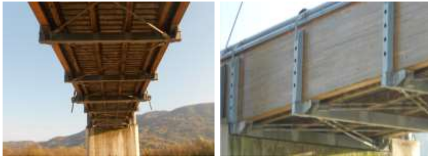
Figure 2.3.7. View of the structural scheme of the “Tesa” footbridge deck.
