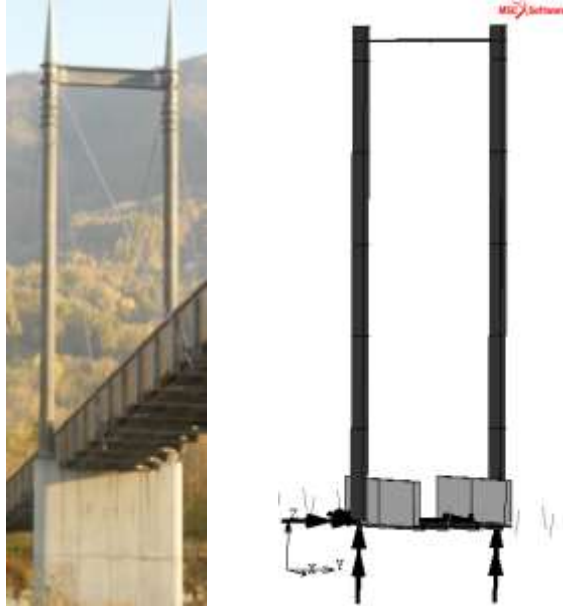
Figure 3.2.3. Detail of the kinematics boundary condition at the base of the pillars. On the left picture from field; on the right the implemented boundary on the numerical model.
