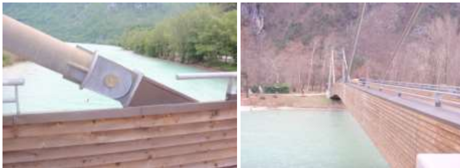
Figure A.1.12. View of the upper protection system of the beam made by copper (left). A detail of the external larch cladding (right).
