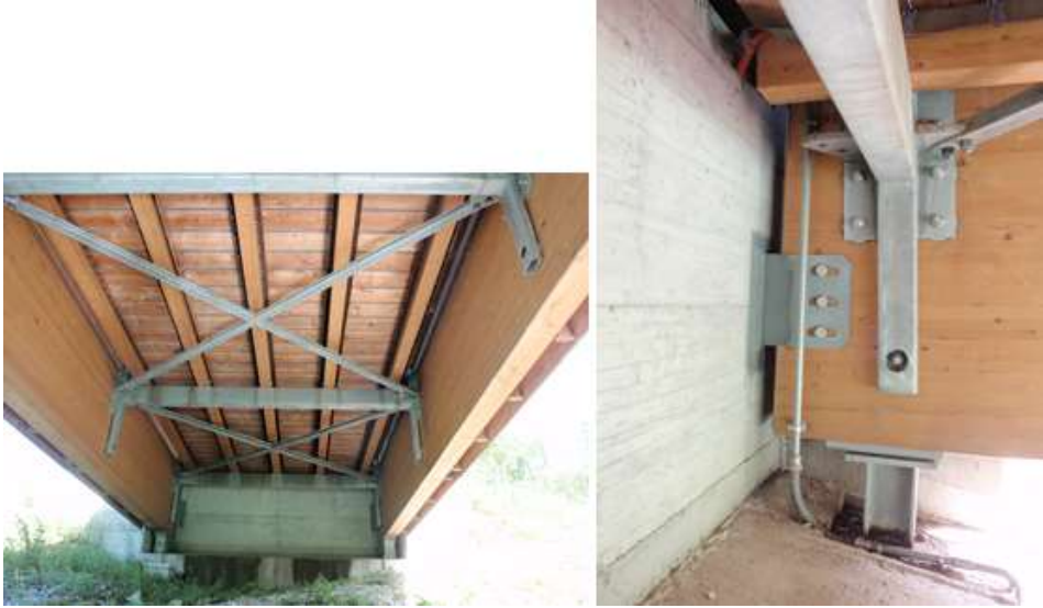
Figure A.1.13. View of the neoprene support.
