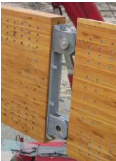
Figure A.2.9. Detail of the joints connection.
