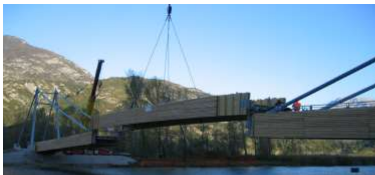
Figure A.1.10. Construction stage: assembling the central section of the footbridge. a) before the assembly; b) during the stage.
