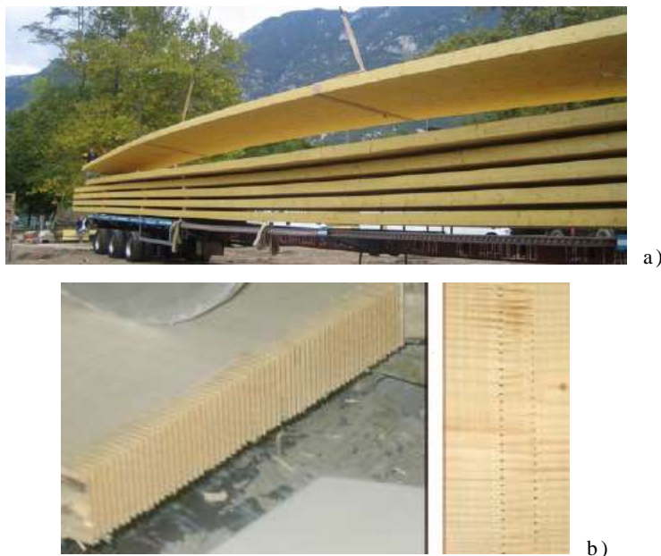
Figure A.1.4. Details of the main GLT beams: a) view during the construction stage; b) details of the joint connection.
