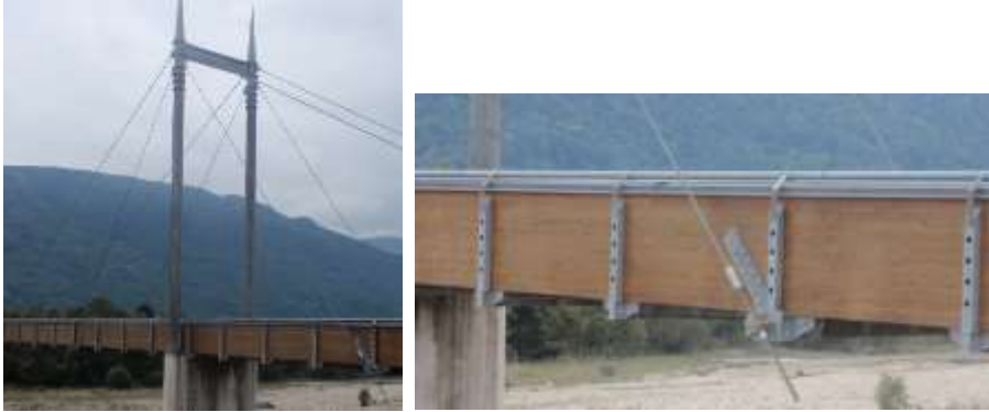
Figure 2.3.6. View of the pillar on the left; detail of the connection between cable and deck on the right.
