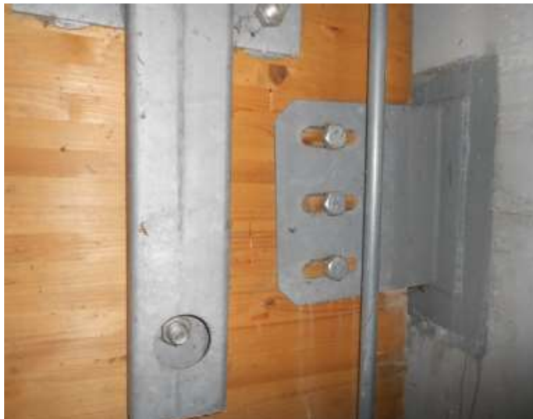
Figure A.1.21. Detail of the connection between the GLT curved beam and the concrete foundation system.
