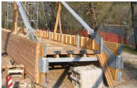
Figure A.1.9. Example of the structural joint connection: connection of the lateral section in correspondence of the steel oblique tubular element.
