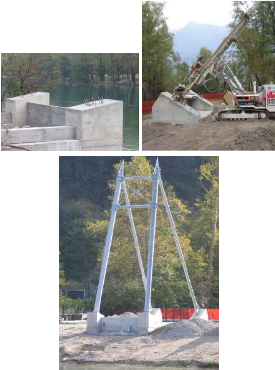
Figure A.1.19. View of the reinforced concrete foundation system.
