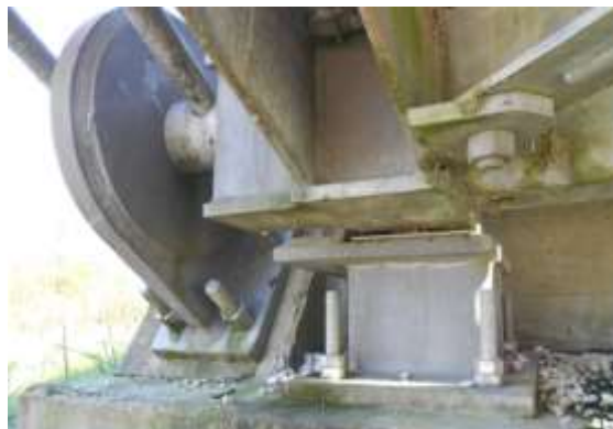
Figure A.2.8. Detail of the neoprene support.
