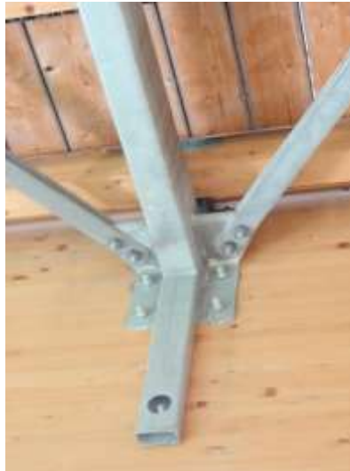
Figure A.1.20. View from above of the walkway. Detail of the H-shape steel element connection with the GLT curved beam.
