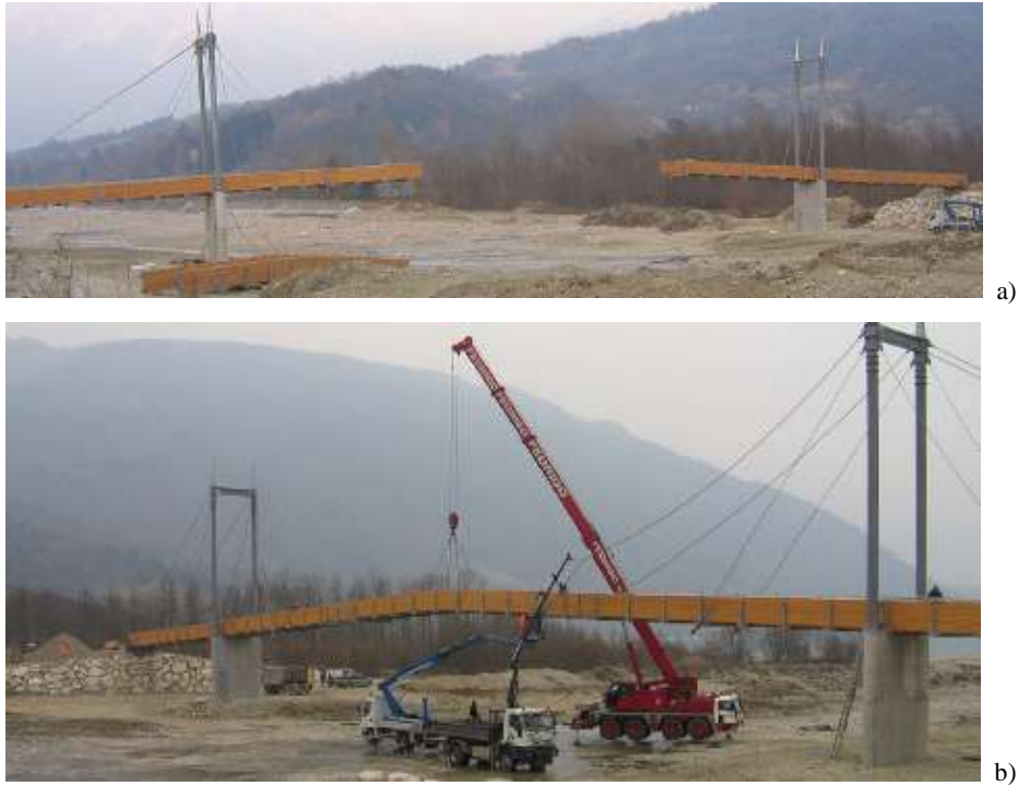
Figure A.2.10. Construction stage: assembling the central section of the footbridge. a) Before the assembly; b) during the stage.
