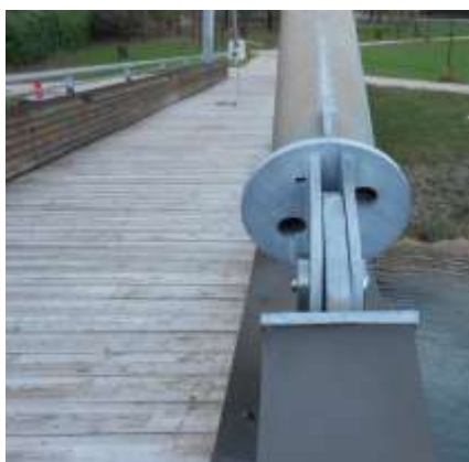
Figure A.1.18. Detail of the structural joint between the GLT curved beam and the oblique steel tubular element.
