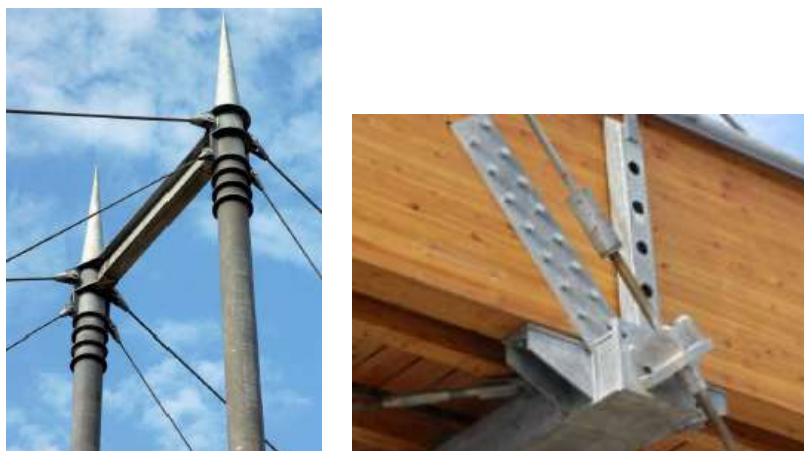
Figure A.2.5. Detail of the joint connection with the steel cables. Connection with antenna (left); connection with the deck (right).
