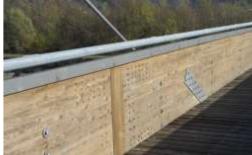
Figure A.2.14. Detail of the upper protection of the main GLT arcuate beams.
