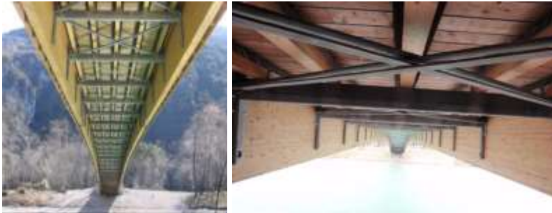
Figure 2.3.3. View from the bottom of the “Trasaghis” footbridge on the left. Zoom on the structural resistant scheme of the deck on the right.
