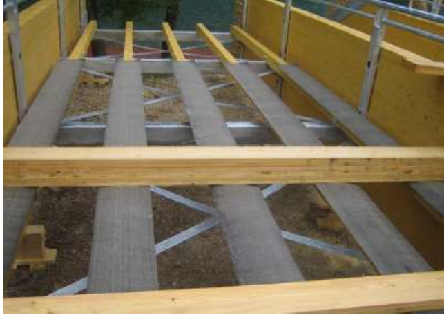
Figure A.1.7. Detail of the walking table during the construction stage.
