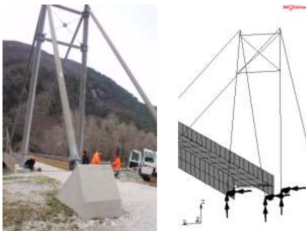
Figure 3.3.3. Detail of the kinematics boundary condition at the base of the stays. On the left picture from field; on the right the implemented boundary on the numerical model.
