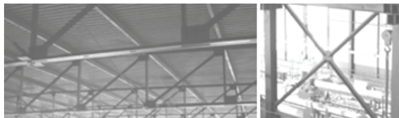
Figure 4.3. Internal 2D Pratt truss (left) and wind-braces (right)
