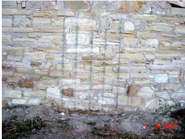
Figure 4.18: Pre-stressing devices used to apply tension in the assembly.
