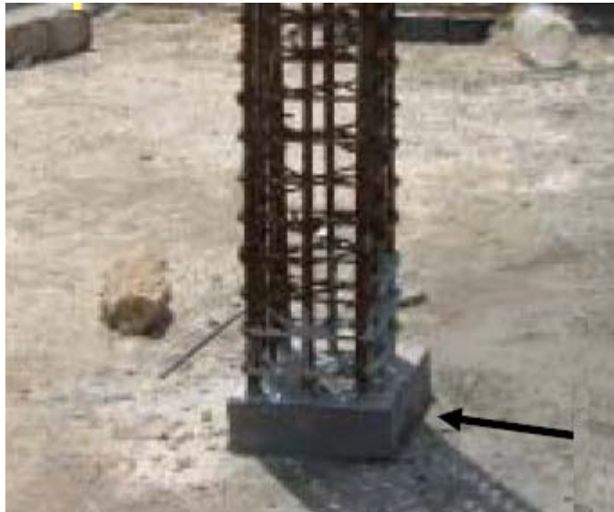
Figure 2.8: Thimble at the basement of columns used for easier framework.
