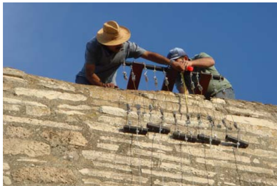
Figure 4.17: SMA wires supported at the rigid base at the top of the pier of the aqueduct.
