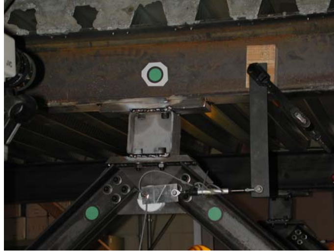
Figure 5.21: Passive HYDE device installed on the Baby-Frame.
