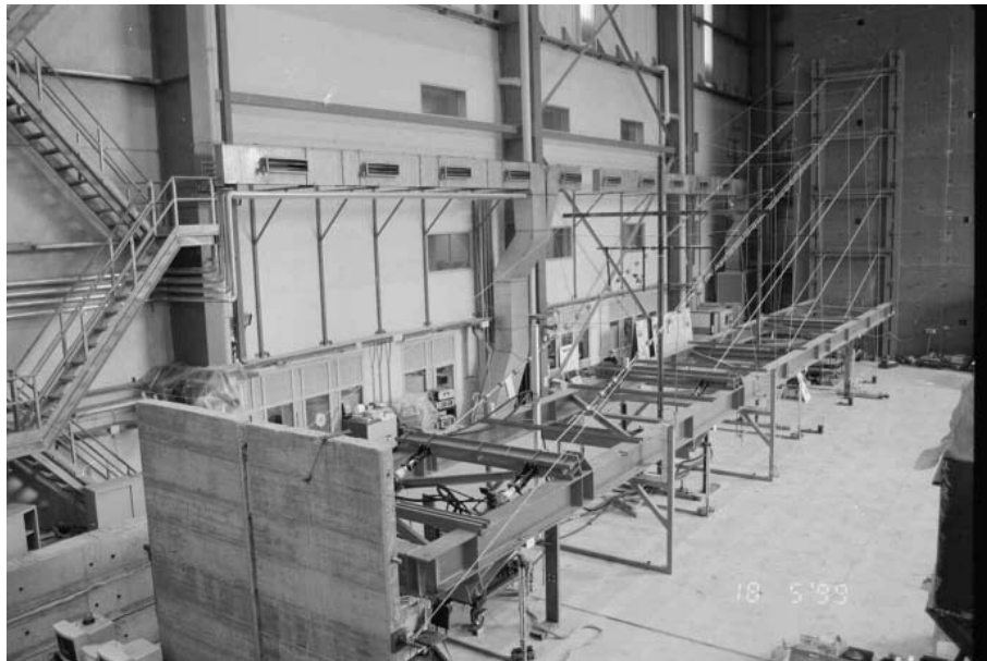
Figure 5.25: Large scale cable-stayed bridge mock-up
