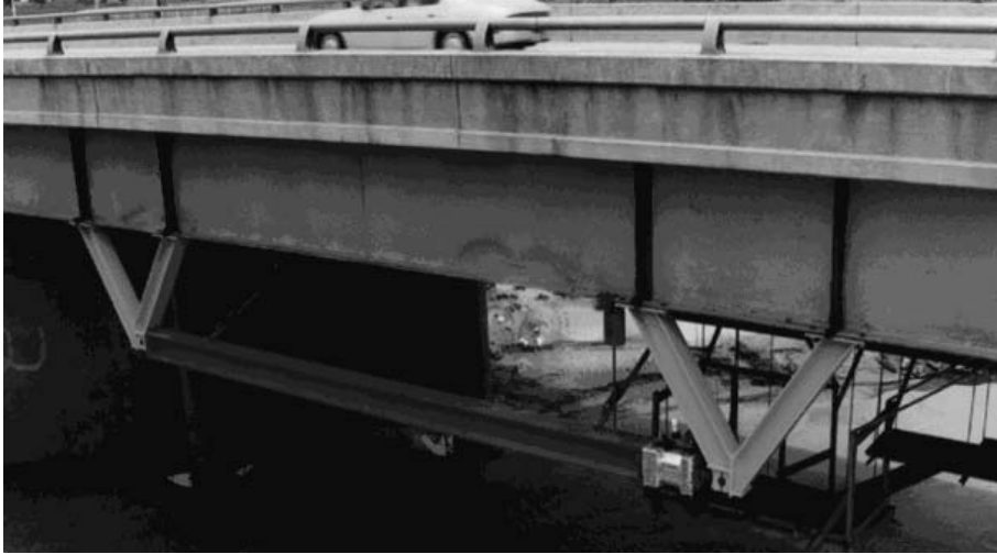
(a) Bridge view
