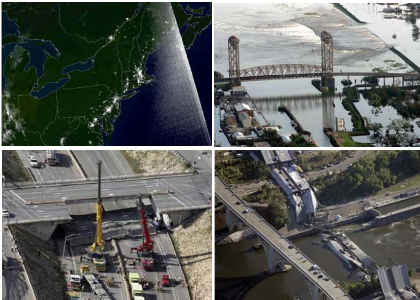
Figure 2.3. From top left to bottom right, the U.S. Northeast Blackout of 2003 (Defence Meteorological Satellite Program), a failed levee in New Orleans during Hurricane Katrina in 2005 (Associated Press), the 2006 collapse of an interstate overpass in Laval, Canada (CCTV News), and the 2007 Collapse of the I35W Bridge in Minneapolis, Minnesota (Minnesota State Department of Transportation).
