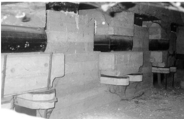
Figura 1-28: Rubber bearings placed between the strip foundation and the building (Scuola Heinrich Pestalozzi di Skopje 1969)
