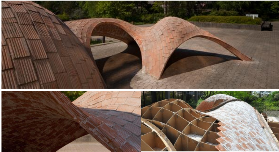
Figure 2.3 – Free-form Catalan Thin-tile vault, project by the Block Research Group, ETH Zurich, ( http://block.arch.ethz.ch/projects/freeform-catalan-thin-tile-vaulting ).
