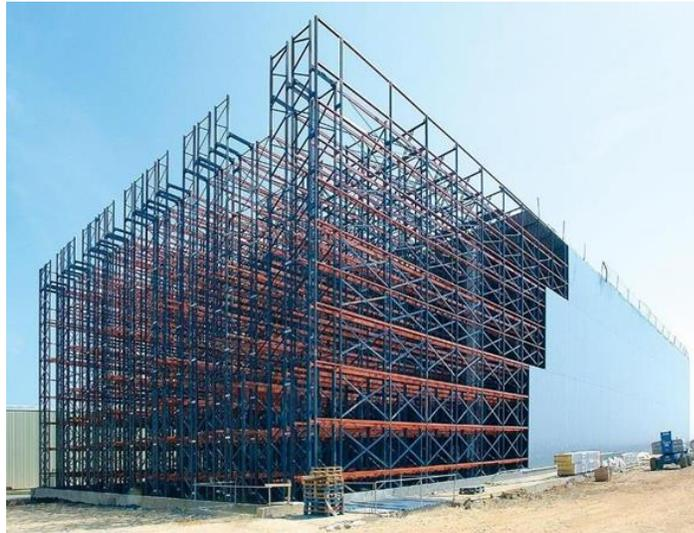
**Figure 1-6. Cladding pallet rack structure.**
