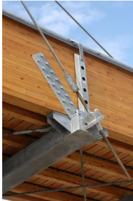
Figure B.4 Detail of the joint connection with deck
