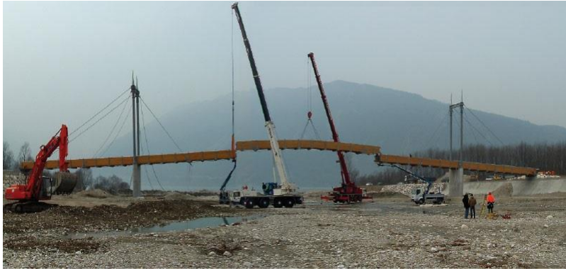
Figure B.7 Construction stage: assembling the central section of the footbridge
